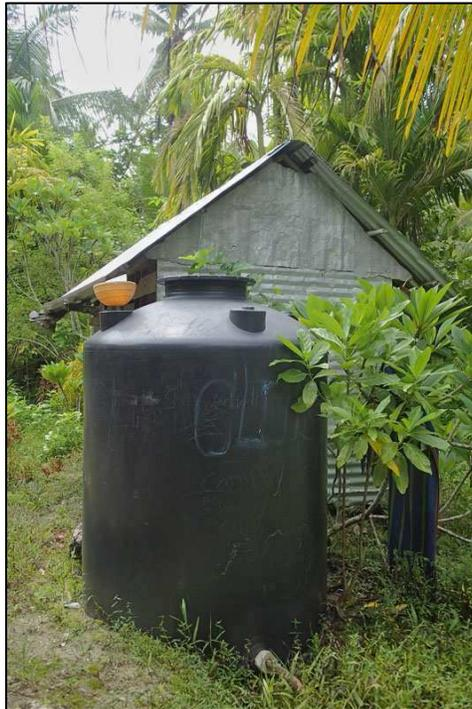
Figure 15 – Photograph of a rainwater catchment storage tank on Ifalik (Photo credit: iREi, 2015)
