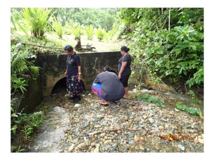
Figure 21. While the community cleared debris from the stream, the culvert appears to be too small to accommodate the fluctuating volume of water flow from streams and is likely to become clogged again.
