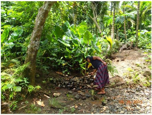
Figure 14. Bernie Mininug adding rocks to a modest retaining wall that prevents the erosion of rich mud from the taro patch which is already starting to thrive. This is an example of Yapese "nature-integrated technology" where people work along with natural processes.
