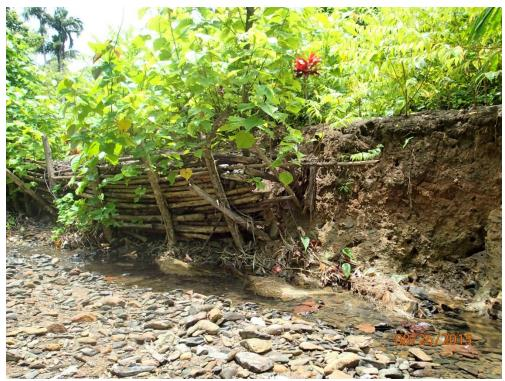
Figure 12. Retaining wall built with small logs and held in place by *Hibiscus* stakes that have since sprouted to form living posts.
