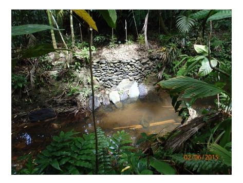
Figure 7. Larger rocks are used where the pressure of flowing water is greatest. Shrubs and trees are then planted along the stabilized stream to help hold the soil.
