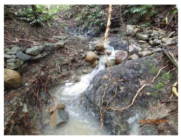
Figure 20. Rockwork was installed to withstand increased water force at curves.
