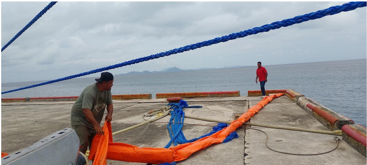
Image 3: 4/20/26: Placement of oil boom on site
