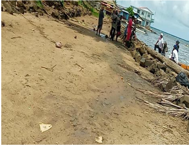
Image 6. Discoloration sandy road/oil carried inland during high-tide
