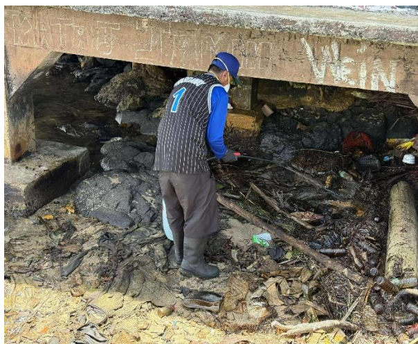
1. Low-pressure washing/collection of oily waste
