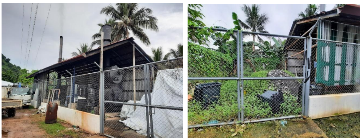
Image 4: Chuuk State Hospital Medical Waste Incinerator
