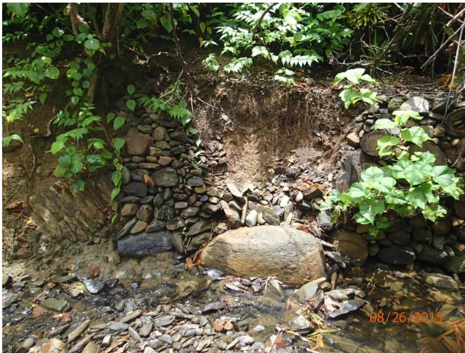
Figure 16. Rock walls built to protect stream bank at a curve where water flow has more force. A portion of the wall has been damaged by heavy water flow following intense rains associated with passing typhoons.
