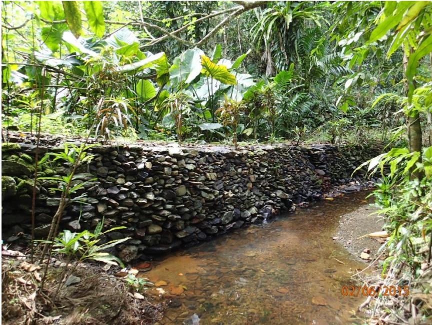
Figure 8. Hand built rock wall prevents stream from washing away rich silts needed to grow taro in taro patch in background. Upland taro patches are now being renovated to replace lower lying coastal taro patches that have been affected by salt water intrusion.
