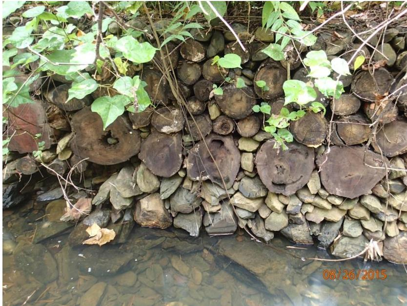
Figure 11. Retaining wall built of rocks and short logs as there were not many large rocks on the site.
