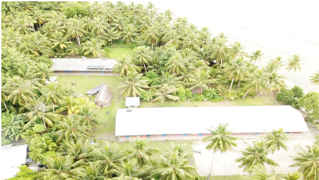
Figure 34. Photo of Lamotrek School and Solar Panels
