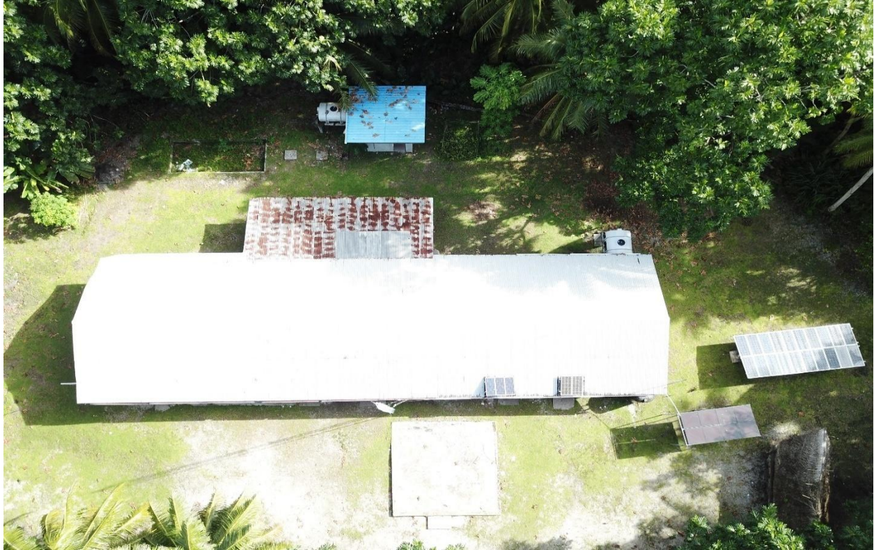
Figure 21. Photo of Woleai Atoll – Falalus Elementary School
