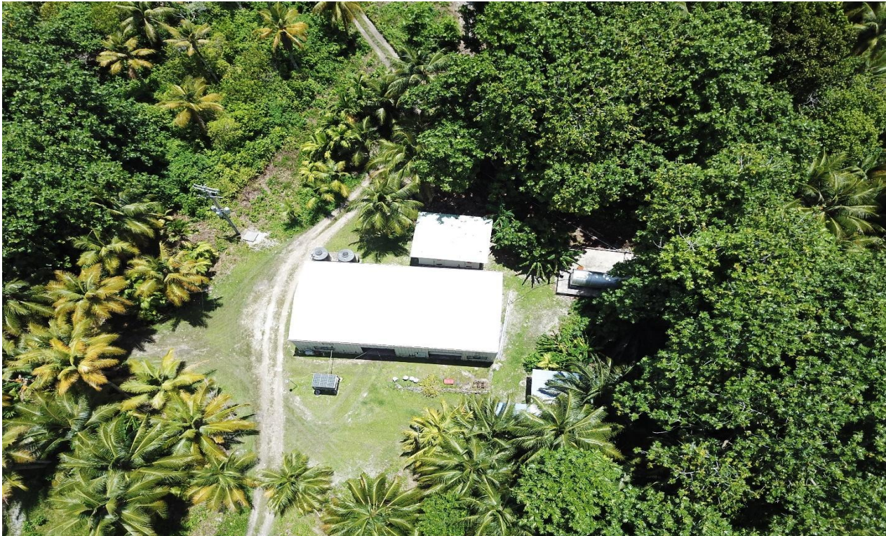
Figure 24. Photo of Woleai Power Plant
