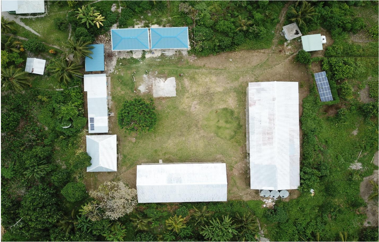
Figure 13. Photo of Fais Atoll School, Library and Solar Panels
