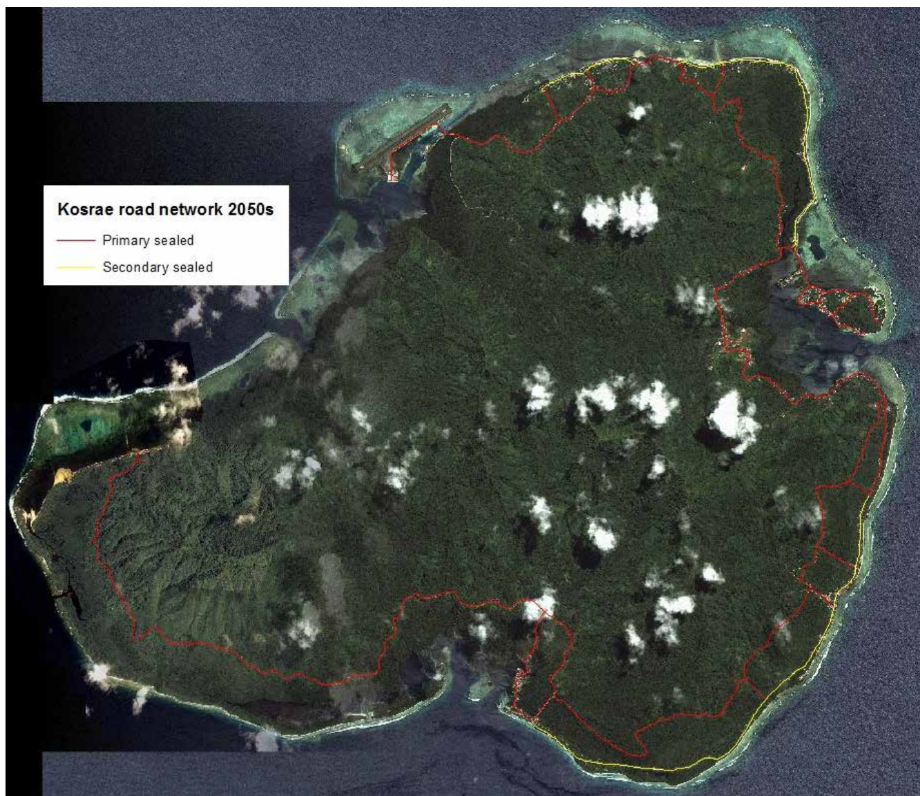
Figure 13: Potential primary and secondary sealed road network on Kosrae by the 2050s. Note: Parts of the secondary road network (current coastal road) may become impassable due to ongoing shoreline change and breaching.
