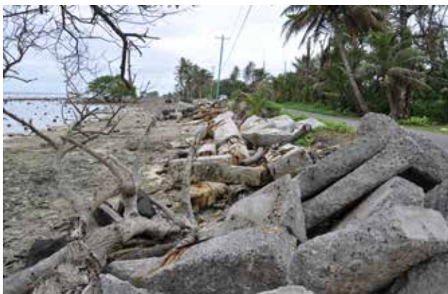
Figure 5: Recent examples of poor development activities that will lead to further coastal hazard-related problems and are not sustainable or effective in the long-term. Top left: Low-lying reclamation for a new laundromat at Tafuyat, Lelu Harbour; Top right: Concrete bag seawall to protect the road at Mosral, Malem; Bottom left: Dumped concrete rubble to attempt to protect the road at Pal, Malem; Bottom right: Access road construction through the mangrove and along the foreshore at Leap, Walung.
